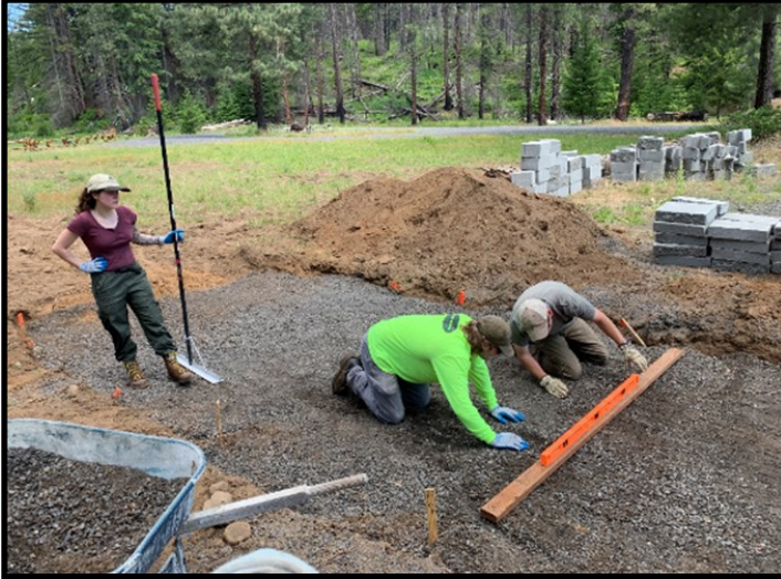
WCC assisting us in grading the pad for the horse ramp
