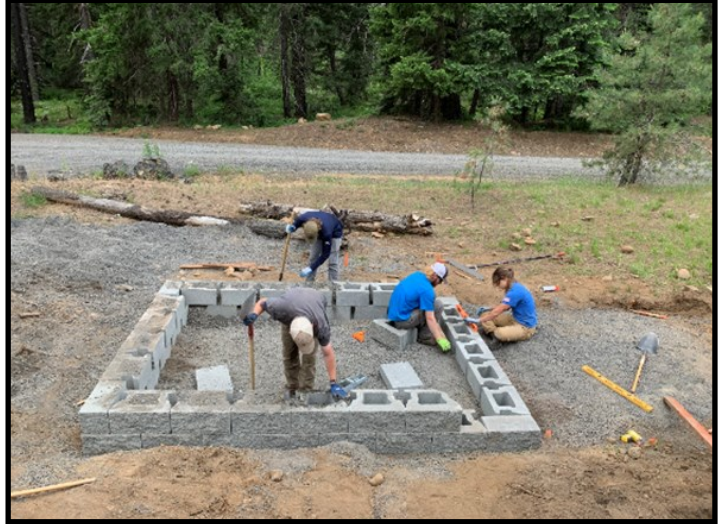
Setting the first couple courses of block for the ramp
